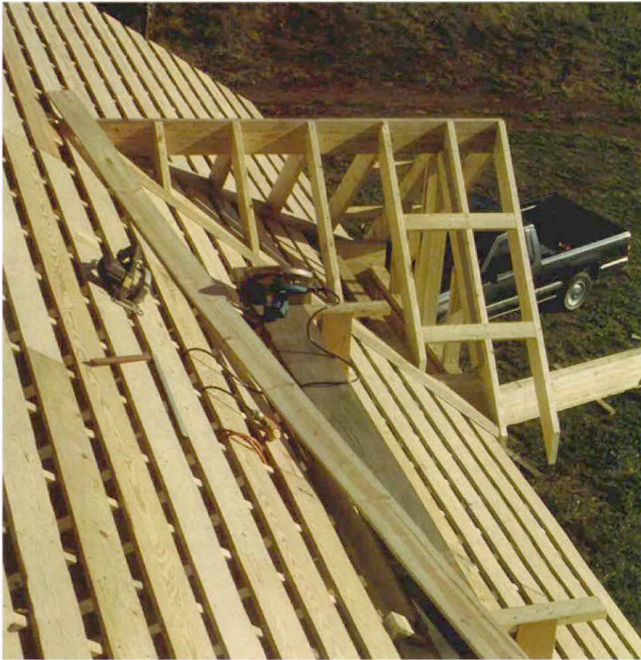
One roof framed on another. A California roof features valley boards that lie flat on the main roof sheathing. As opposed to a valley rafter, there's only one set of jack rafters to cut and one cheek-cut setting on the circular saw.
