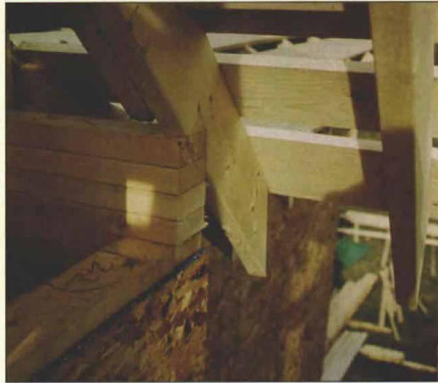
Additional top plates provide bearing for the kickout's 2x6 rafters while picking them up enough to line up the fascia boards.
